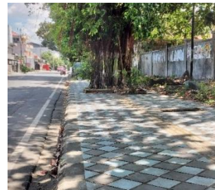
Figure 6. A Tree In The Middle Of The Sidewalk Presents A Sidewalk Obstacle.
